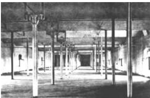
Figura 1.6 Fábrica de Farinha Marshall, Benyon & Bagé. Ditheringthorpe – 1796
