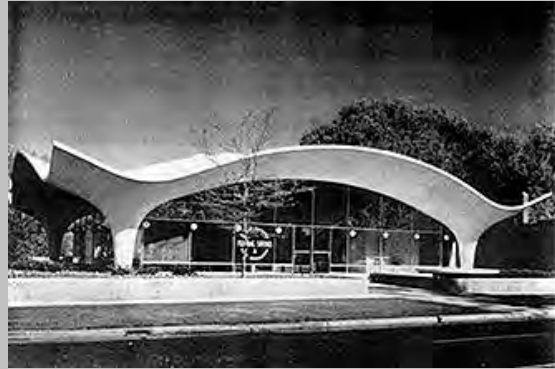
Figura 9.1.22 - Mount Clemens Federal Savings & Loan Association, M. Clemens, Michigan. Meathe, Kessler & Associates, Inc. Architectural Forum , outubro de 1961, p.99.
