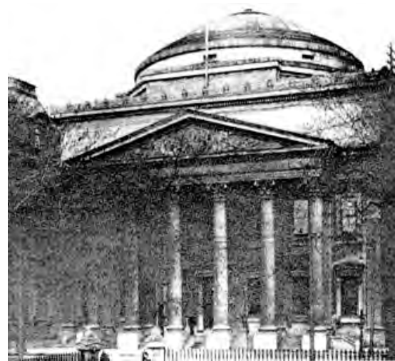
Figura 8.3.3 - Bank of Montreal, Montreal. Mc Kim, Mead & White. Architectural Record , janeiro de 1909, p.11.
