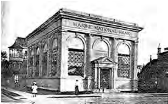
Figura 4.7.13 - Marine National Bank, Wildwood, New Jersey. Henry A. Macomb. Architectural Record , janeiro, 1909, p. 54.
