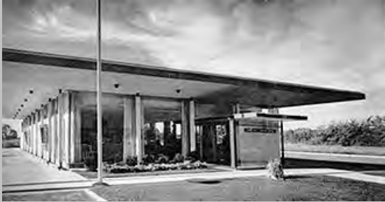
Figura 9.1.13 - Manufacturers' National Bank of Detroit, Dearborn Township, Michigan. Louis G. Redstone. Architectural Record , janeiro de 1961, p.110.
