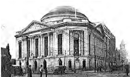
Figura 8.3.5 - Cleveland Trust Company, Cleveland, Ohio. Geo. B. Post & Sons. Architectural Record , janeiro de 1909, p.15.
