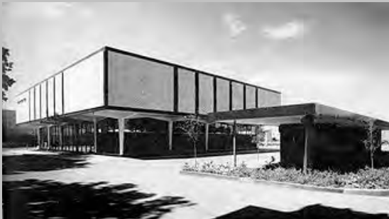
Figura 9.1.19 - First National Bank, San Angelo, Texas. The Office of George Pierce. Architectural Record , janeiro de 1964, p.131.
