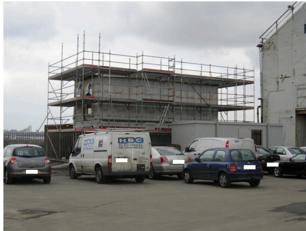
Figure 64: Boxes with scaffolding outside the factory are the showroom
