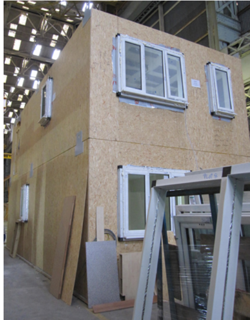
Figure 56: Prototype at the factory: two boxes combined vertically
