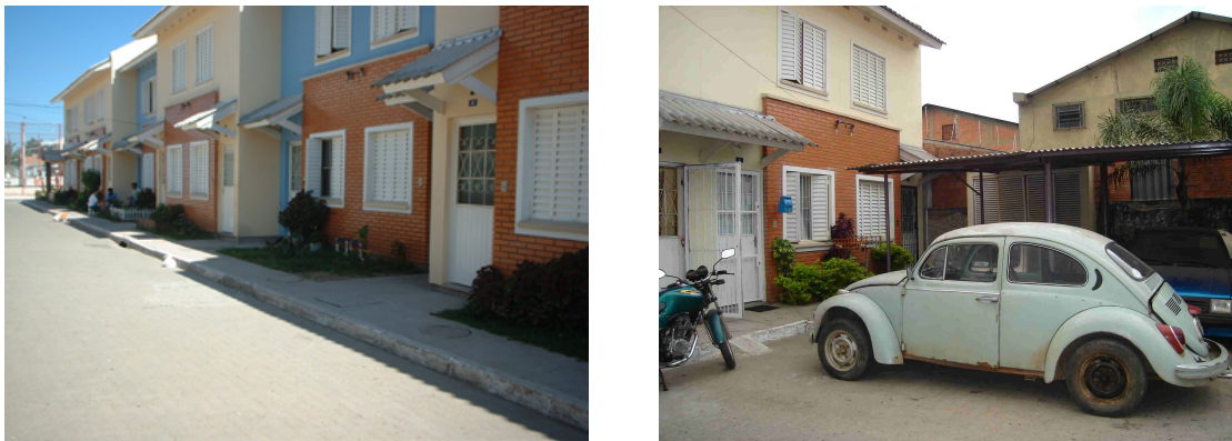
Figure 1: Example of personalisations informally carried out by householders (source: Miron, 2008)
