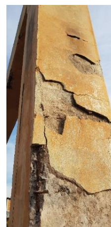
Figura 32 – Pilar 10, face Norte
