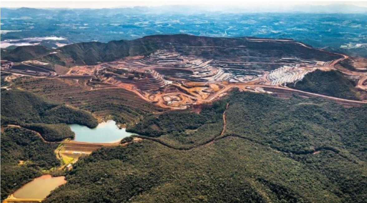
Figure 6: Tamanduá “dry” stacking facility, probably the largest dry stacking in Brazil (VALE S.A., 2019).
