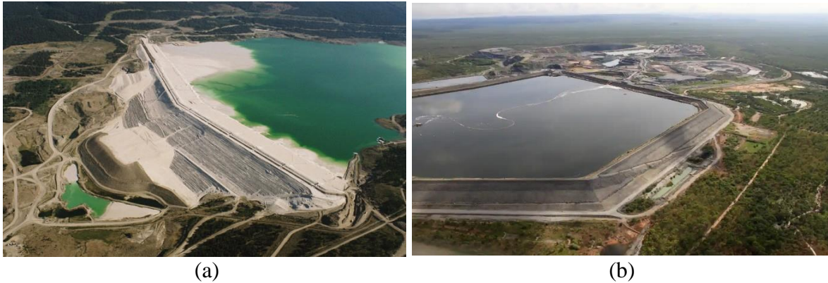
Figure 3: Tailings storage facilities: a) Cross-valley impoundment (Berger, 2018); and b) ring-dike design (Davidson, H - The Guardian, 2019).
