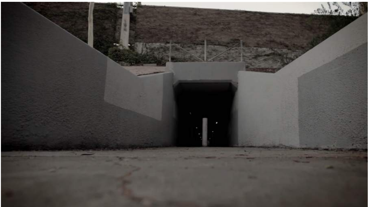
Figure 10 – View of the underpass near Tricia's house.
