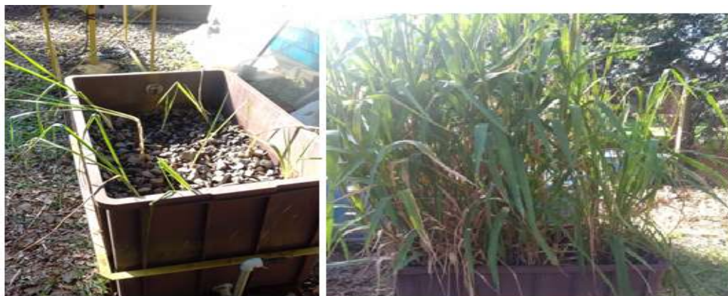
Figure 3: Construction of subsurface vertical flow vertical constructed wetland biomass (VFCW) and production of Hymenachne grumosa biomass.
