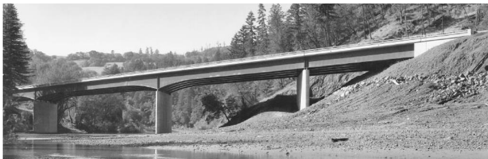
Figura 7. Eel River Bridge (ROOT, 1999)
