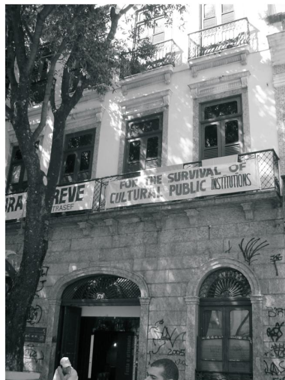
40.3-Fachada frontal CNFCP.
