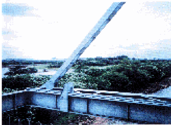
Fig. 4.23 - View of the dam structure in the area of the dam, showing the concrete structure and the concrete beam.
