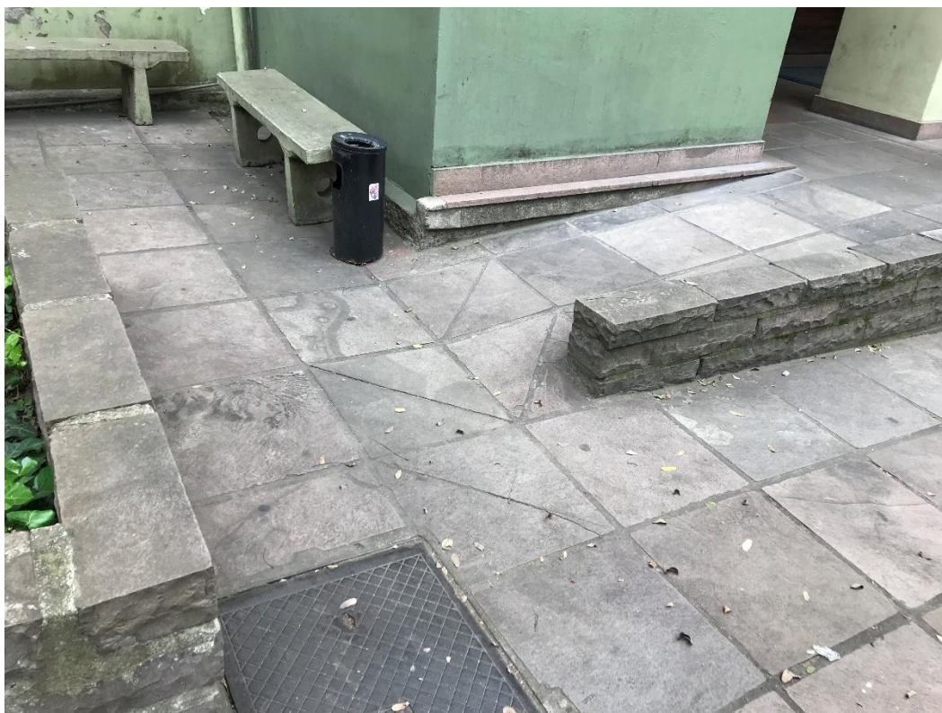
Figura 35 - Rampa principal FCE
