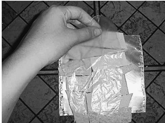
Fig. 7. Assembly of the hot melt second layer.
